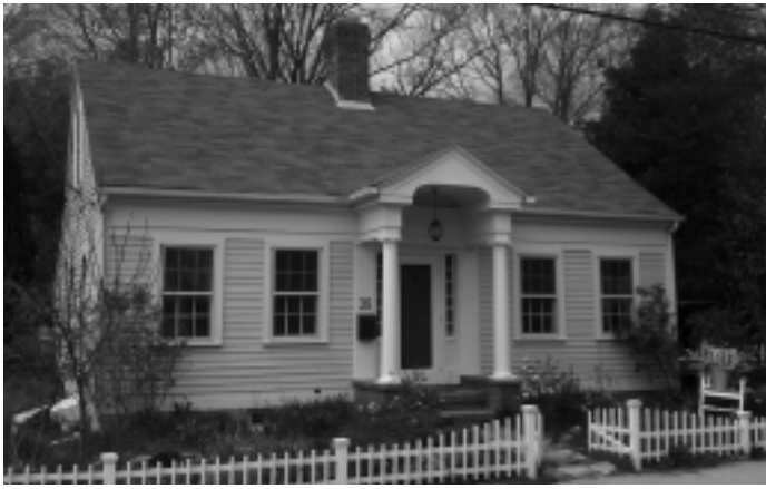
This 1844 historic district home has seen relatively few exterior changes to its classic Cape form since it was built. An exception is the unusual formal portico entry - a Greek Revival touch which was added in the 1920's.
