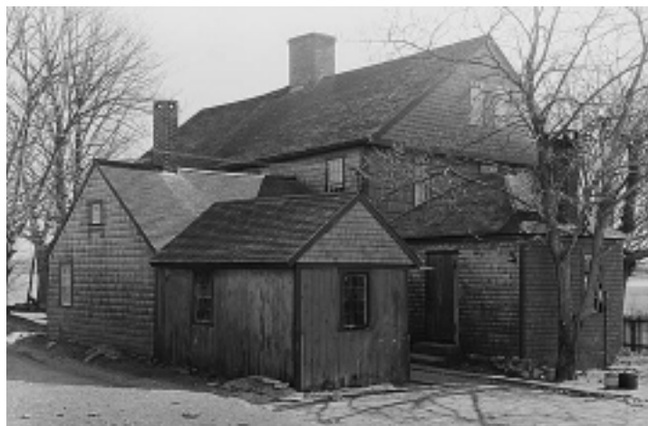
Photo of the rear view of the historic Stanton-Davis Homestead
