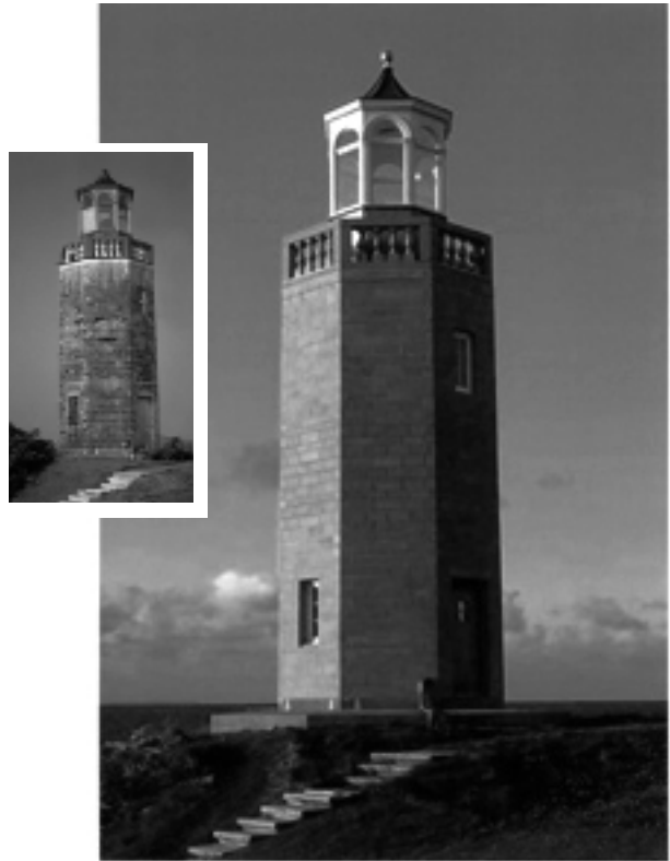
The Avery Point Lighthouse in August 2000 (inset) and after careful & extensive renovations in December 2005 above.
